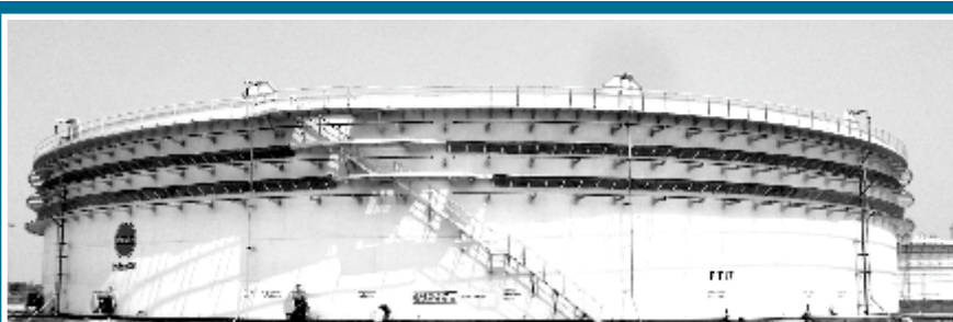
Crude Oil Storage Tank at IOCL, Paradip
