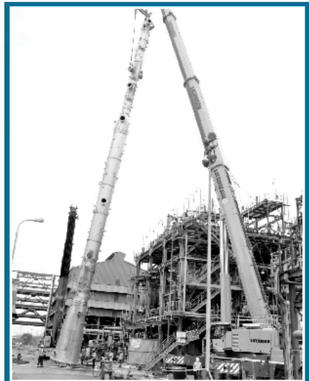
Column erection work at Visakh Refinery, HPCL
