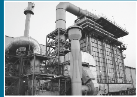
Radiant Heater at MCPI, Haldia
