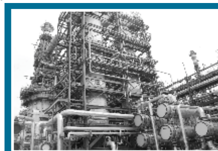
Piping and equipment work of NHT / CCR Unit at Visakh Refinery, HPCL
