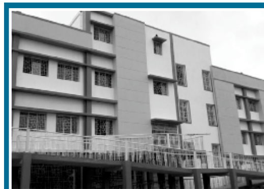
Construction of Multipurpose Cyclone Shelters under National Cyclone Risk Mitigation Project (NCRMP-II) at different locations in West Bengal
